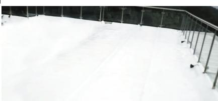
Water Proofing membranes are typically installed using mechanical fasteners and plates placed along the edge of the membrane and fastened through the membrane and into the roof decking. Adjoining sheets of membrane are overlapped, covering the fasteners and plates, and joined together with a minimum 40mm wide hot air weld.
